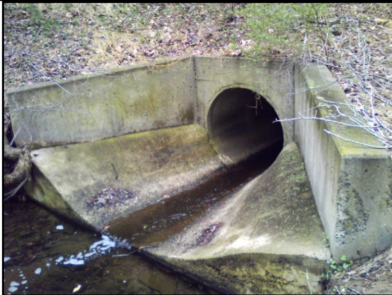
Photograph 12: View of an outfall delivering stormwater runoff from I-287 directly to TR4-1.
