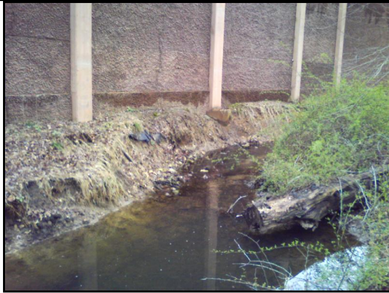
Photograph 7: View looking upstream at TR4-1 showing erosion along an outer bend exposing structural support of the I-287 sound barrier wall.
