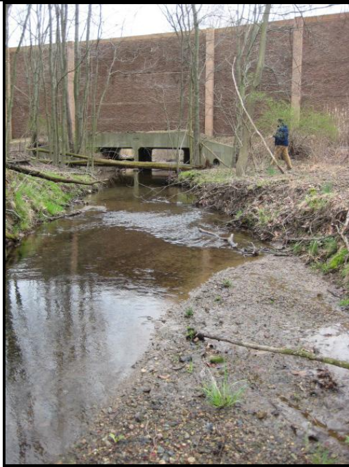
Photograph 1: View looking downstream at I-287 crossing over MS3. The culvert is typical of I-287 stream crossings.
