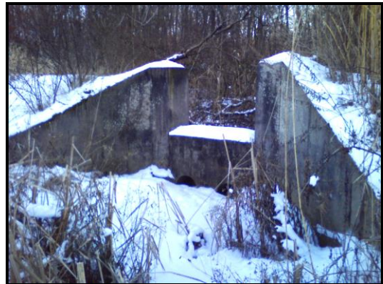
View of outlet structure from Basin 5.
